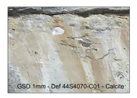
Upstream & downstream orthoplans of the dam facings (Switzerland), August 2015. Work done from 5000 aerial photographs (by facing) made by the AirX3 company with its drone Falcon 8 and a 1mm resolution. Structural analysis of the disorders (cracks, vegetation, infiltration, joints, calcite etc.) and location made on orthoplans by Drones Imaging.
